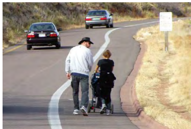
Although not ideal, the “walkable shoulder” may be an option in rural areas where traffic volume is low.
