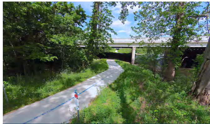
Concrete Fall Creek Trail - Indianapolis, IN
