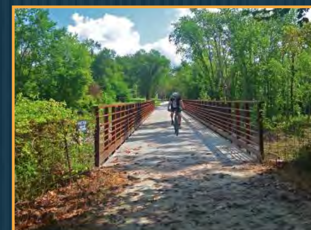
Outside of bridge structures, much of the trail surface is crushed and finely packed gravel. This provides minimal resistance for bikers and an ideal surface for runners or walkers due to the lower impact than asphalt or other paved surfaces.
