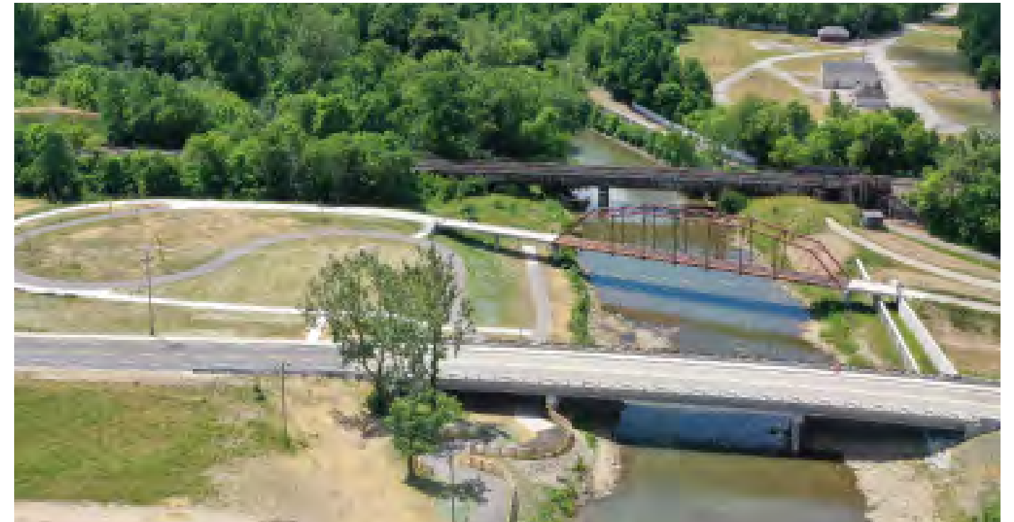
Kitselman Trailhead - Refurbished INDOT bridge for pedestrian use (Kitselman Trail - Muncie, IN)
