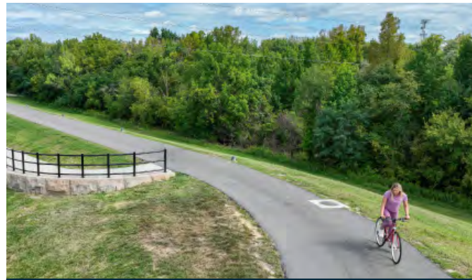
Asphalt Silver Creek Trail - New Albany, IN
