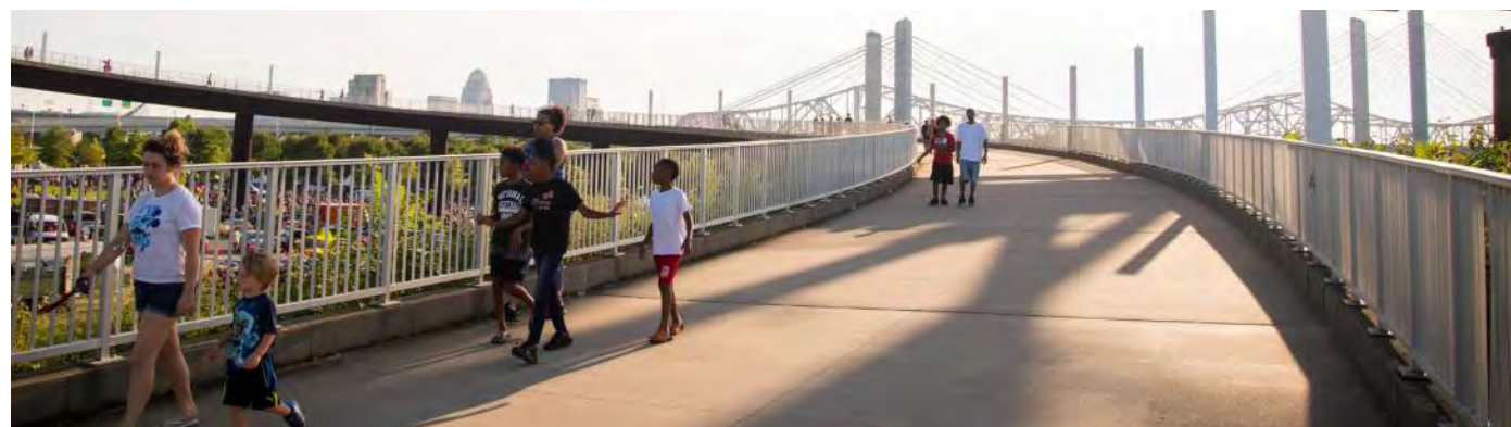
The Big4 pedestrian bridge in Jeffersonville, Indiana connects the Ohio River Greenway to Louisville, Kentucky.
